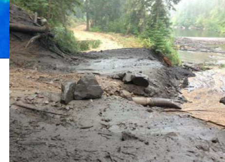
Extreme Weather-related Water Hazards
